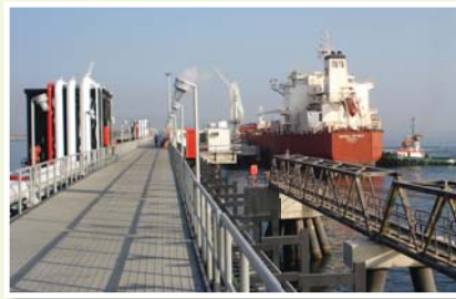
Topaz Engineering completes berth construction
